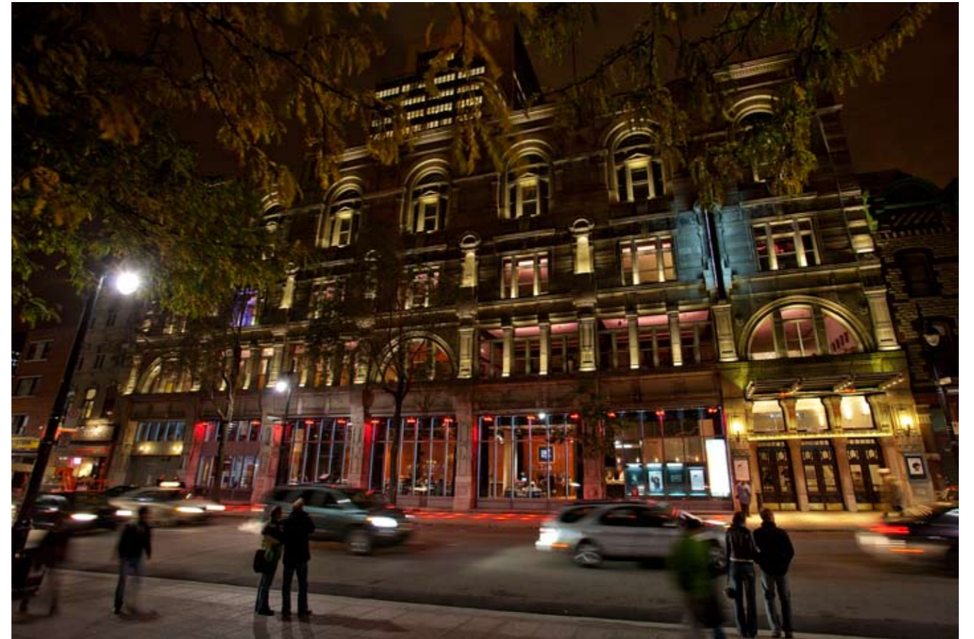
Canada, Montréal Monument National, Quartier des Spectacles To honour the National Monument, 160 LED light fittings made by Schröder have been developed in compliance with the lighting plan of Montréal and the city's commitment to environmental responsibility. LEDs bring this 19th century building in line with the codes of the 21st; the red colour reminds us that this is the aptly named 'Quartier des Spectacles'.
