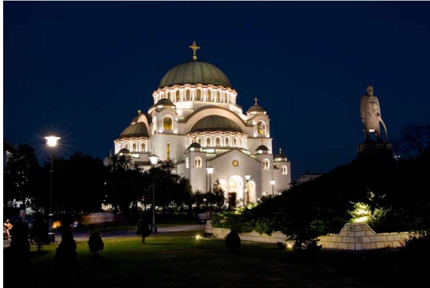
Serbia, Belgrade St. Sava Church To light this prestigious building and create a sumptuous visual effect, 1300 floodlights were needed, of which 600 are in LED version. A jewel box of lights for St Sava Orthodox Cathedral (Belgrade).
