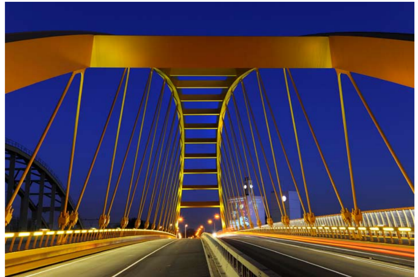
Netherlands, Utrecht Hogeweidebrug A multimodal bridge fitted with 480 linear ground-recessed LED fittings, pairing functionality and stunning visual impact. Ingeniously, it was designed to be 'plug & play' and incorporates dimming technology.
