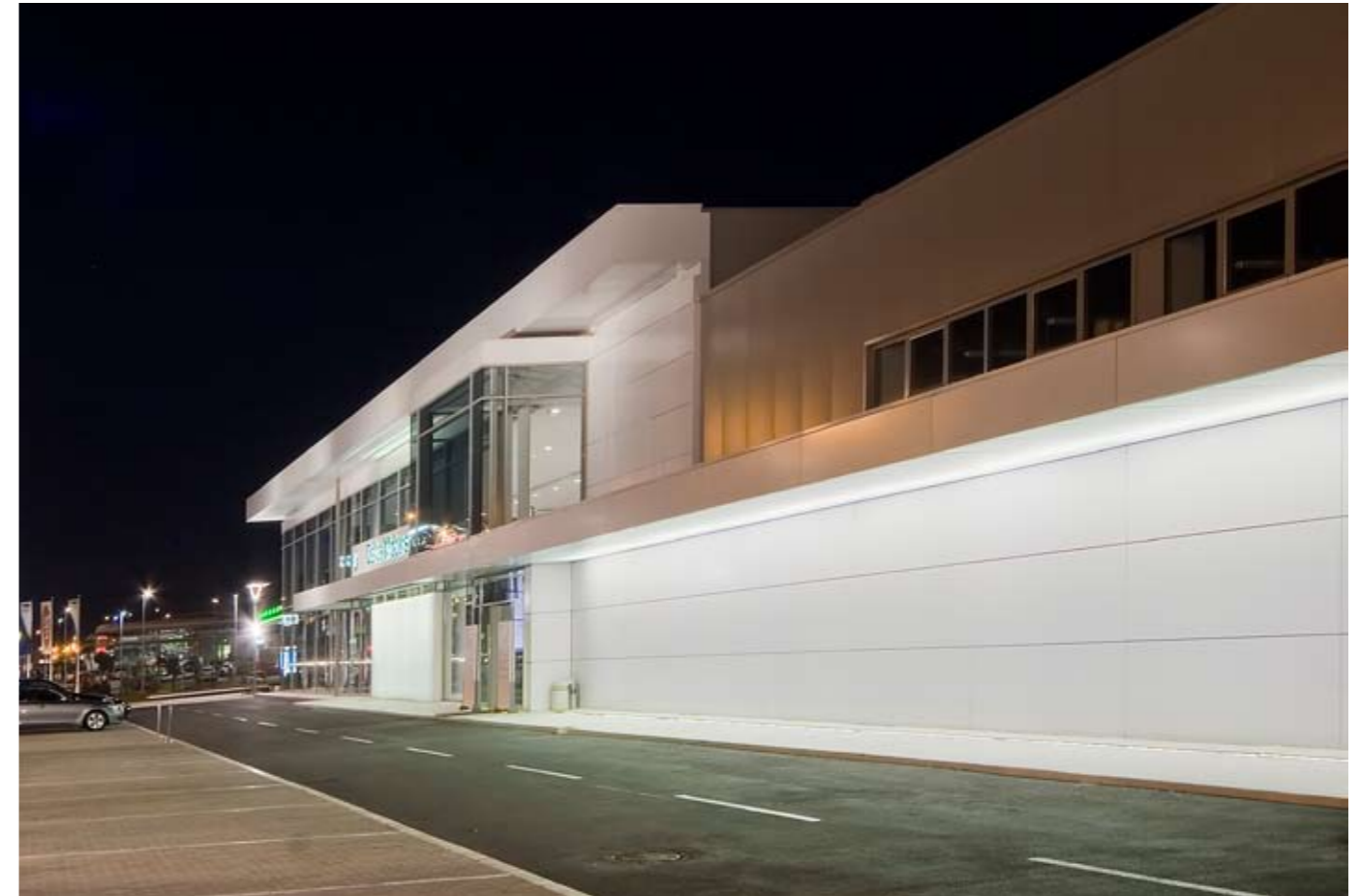
Serbia, Belgrade BMW Showroom LED technology at the service of a leading car maker. What do they have in common? Being made to last, and daring to use innovative designs.
